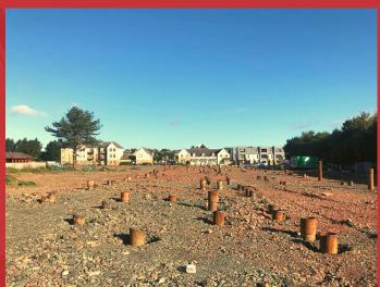
NPL were subcontracted to design, supply and install steel tubular piles for a new low carbon, Eco-friendly, residential area just outside Edinburgh city Centre. The project would see over 120 new energy efficient homes, made up of 1, 2 and 3 bedroom apartments.
