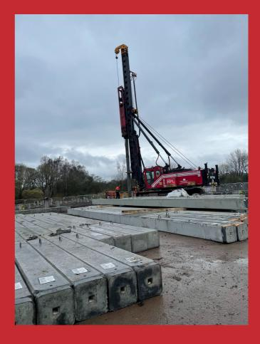
NPL were subcontracted to design, supply and install structural precast piles for the new residential road along Frankfield Loch, Stepps, Glasgow. The new road will replace the old Loch rd, which previously collapsed, providing further access to the new build estate just off the main road, Stepps.
