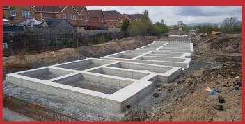
NPL were contracted to design, supply, and install precast concrete piles and Groundbeam package for a residential development on Etna Road in Falkirk. The project was completed in 5 phases and consisted of housing and blocks of flats.
